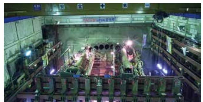
Photo 1 Pipe roofing scene
