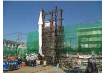
Photo 1 Underground RC diaphragm wall construction conditions
