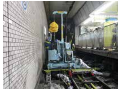
Photo 2 Ground improvement construction from within the station
