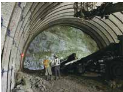
Photo 2 Projection of a photo of the Cutting Face
