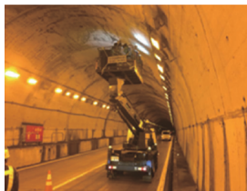
Photo 3 Inspection by close visual inspection
