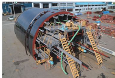
Photo 1 Panoramic view of continuous concrete pouring system using extending/retraction-type hose
