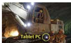
Fig. 3 Using the System at Construction Site
