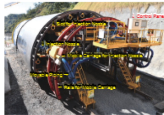
Photo 1 Automatic Concrete Lining System
