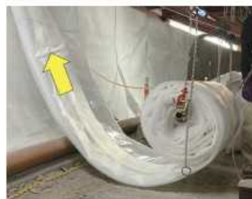
Photo 1 Rolled Waterproof Sheet (pulling up)
