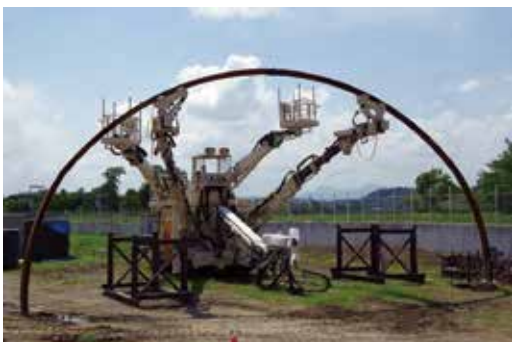
Fig. 2 Photo from the Front of a Support Erecting Robot
