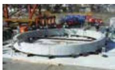
Photo 1 Assembly of segments above ground
