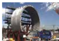
Photo 3 Assembly of 4 rings completed
