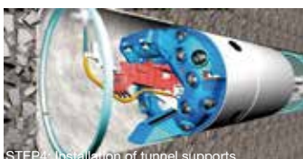
STEP4: Installation of tunnel supports
